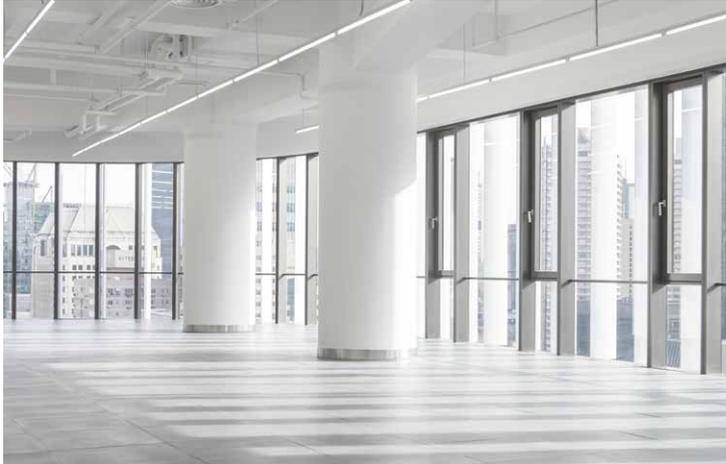
A traditional landlord finished product including: raised floors, suspended ceilings (unless offering exposed services), lighting, fire detection services, heating, ventilation and air conditioning to the standardised building planning grid and occupancy density.
